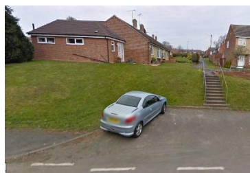
Footpath on the north side ends and pedestrians must take the steps
