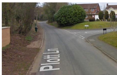
Footpath on the south side (left of frame) ends abruptly
